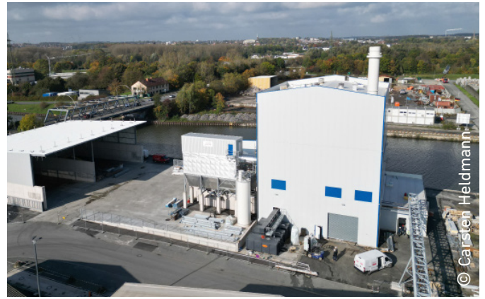
Biomass heating plant under construction.
